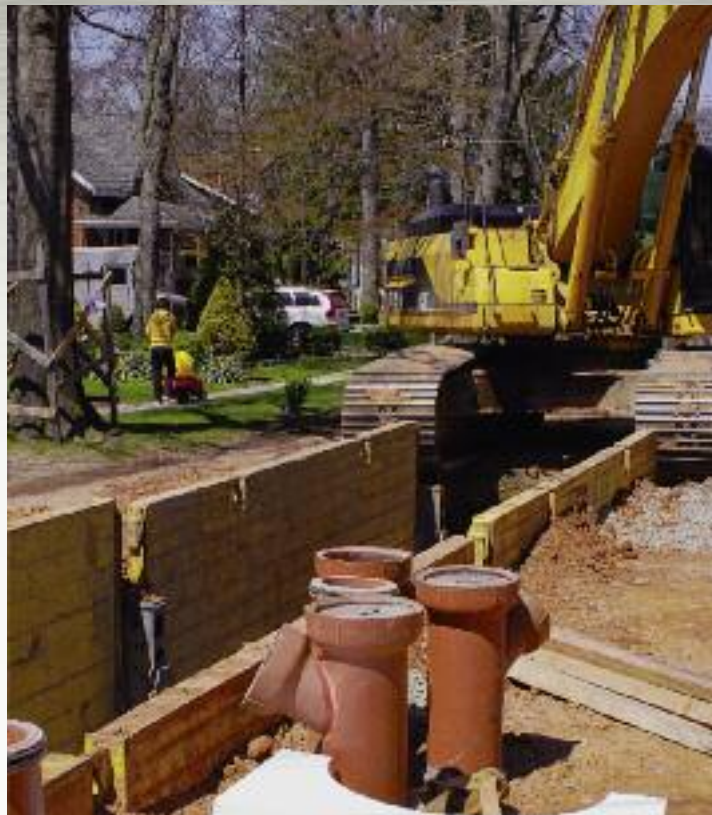
Neighborhood friendly Slide Rail System in action within a Staten Island community.
